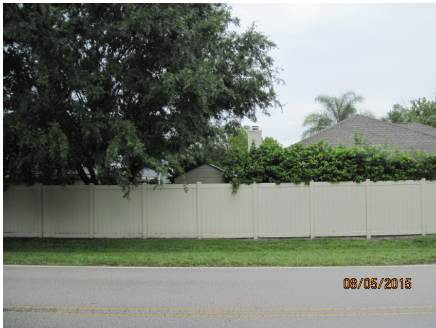
Existing single family across Flynn Road
